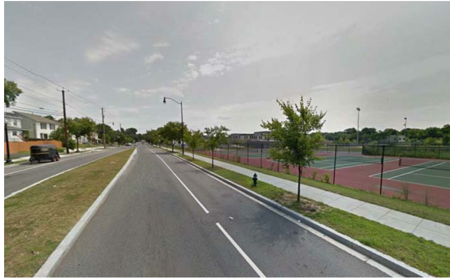
1 VIEW EAST DOWN NANNIE HELEN BURROUGHS AVE NE
